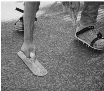
Trowel the sprayed Spray Texture Mix to achieve the desired texture.
