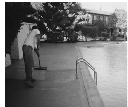
Apply two coats of Concrete Colorcoat using a 1/2 - 3/4" nap roller.
