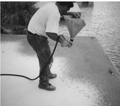
Spray the Ultra Surface Spray Texture Mix using a hopper gun sprayer.
