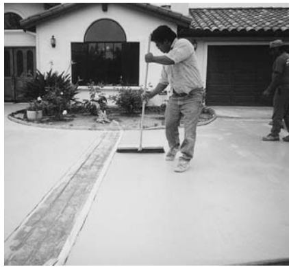
Apply a Fine Broom Finish or Swirl Pattern Finish over the dry Squeegee/Bond Coat.
